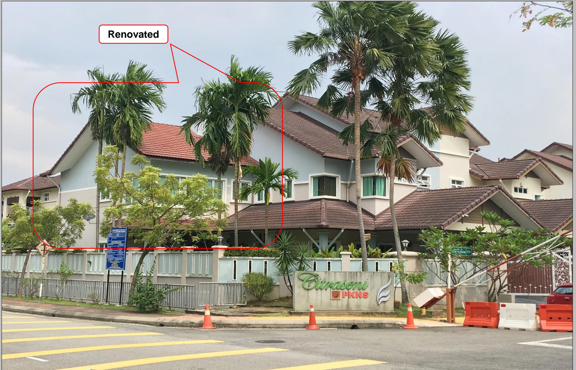
70 Units Double Storey Semi-D House, Section 7, Shah Alam
