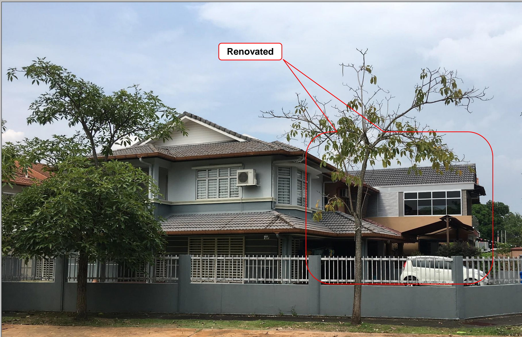
119 Units Double Storey Terrace House, Sec 24, Shah Alam
